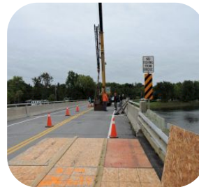
Figure 2: Crane being set up to lower rock to walleye spawning bed from a bridge. (Plywood protects the road.)
