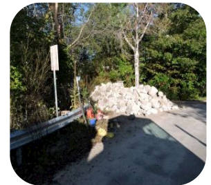
Figure 3: Clean, washed rock is stockpiled before being loaded onto a crane bucket to lower into the spawning bed.
