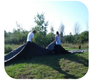
Figure 4: Adding the floats and chains to a new silt curtain.
