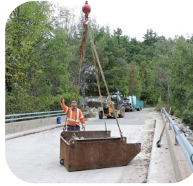
Figure 6: Loader is bringing rock from a pile to place into crane bucket.
